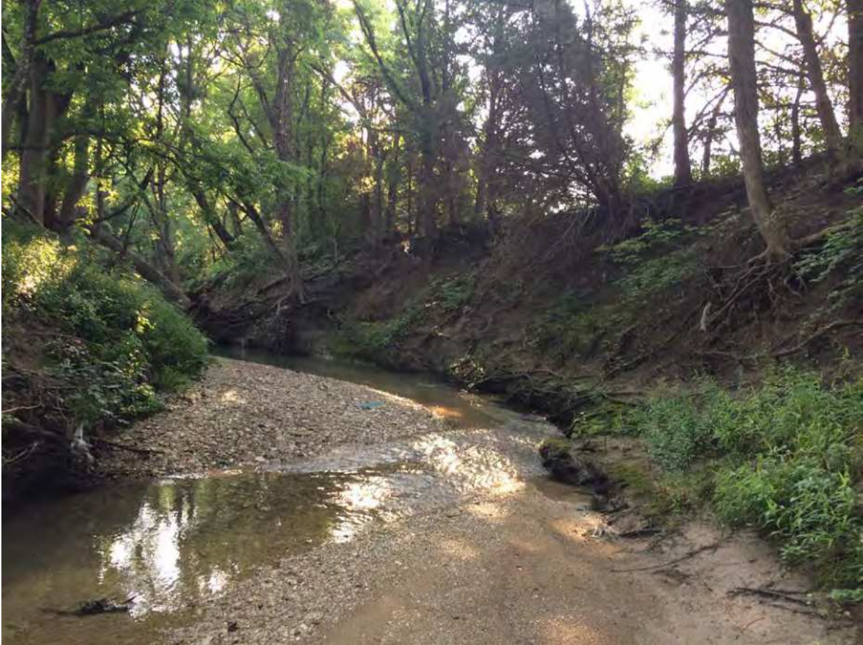
Bank erosion in the outer bend, and aggradation in the inner bend.
